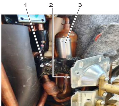
Figure 3-16: Removing the expansion valve
